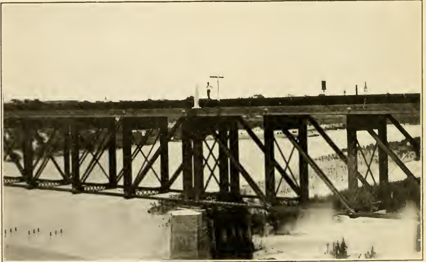
VIEW OF MONUMENT LOOKING DOWN STREAM, TAKEN FROM OLD BRIDGE.
